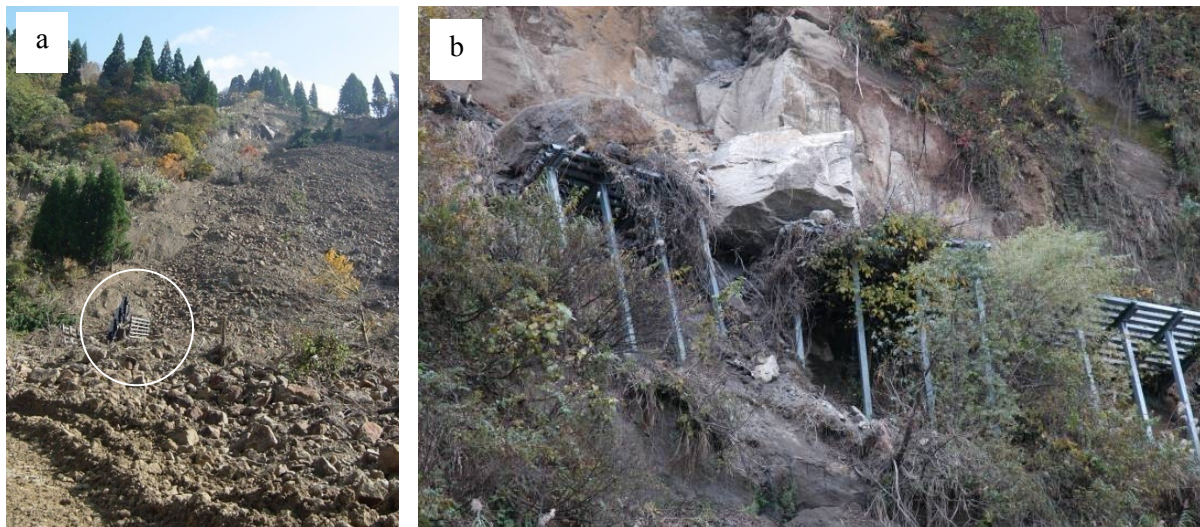
Fig. 63. (a, b) Examples showing damaged snow fences during Chuetsu earthquake in Niigata (M6.8, 23 October 2004).
